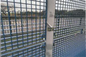
Finding: There is/are finger entrapments in the panels and Action: Monitor - No remedial work recommended the item fails to meet the requirements of BS EN 15312
