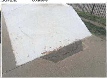
Finding: The riding surface of the ramp has some damage Action: Repair as required apparent
