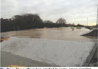
Finding: The surface has eroded in some areas expsing large rocks and may be slippery in wet conditions
