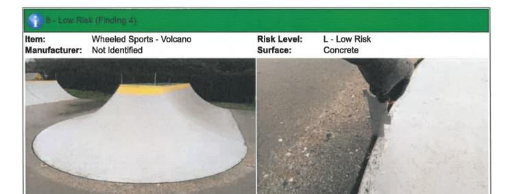
Finding: Height differences between the riding surfaces should not be greater than 3mm to meet the requirements of between the joints do not exceed 3mm BS EN 14974
