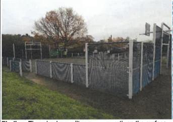
Finding: There is algae, silt or moss growth on the surface Action: Clean and treat appropriately resulting in slippery conditions
