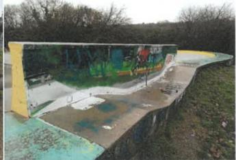
Finding: The adjacent rolling surface does not meet with the **Action**: Monitor - No remedial work recommended requirements of BS EN 14974
