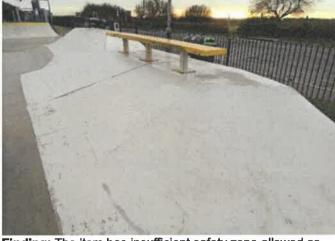
Finding: The item has insufficient safety zone allowed as required by BS EN 14974. This should equal at least 2.0 metres on most items.
