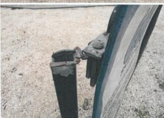
Finding: A section of fence is damaged and unsecured
