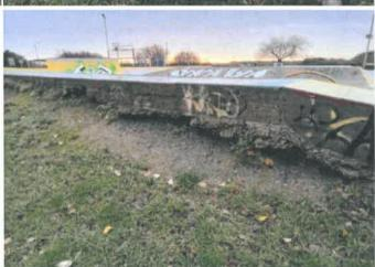
**Finding:** The surface has eroded in some areas exposing the concrete foundations
