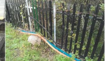
Finding: The fence is severely damaged in places Action: Repair or replace all affected sections
