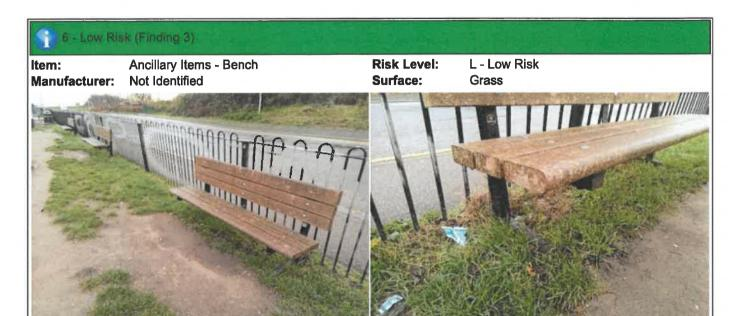
Finding: The paintwork on this item has been damaged or Action: Treat affected areas and repaint worn exposing the metal underneath which is rusting / corroding
